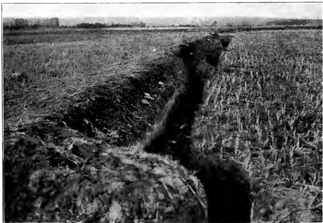
GERMAN TRENCH IN PRACTICE, Showing the traverses.
